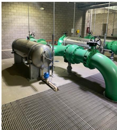
Figure 4 Forsta H18-LP180 Filters at Yucaipa Water Treatment Plant
