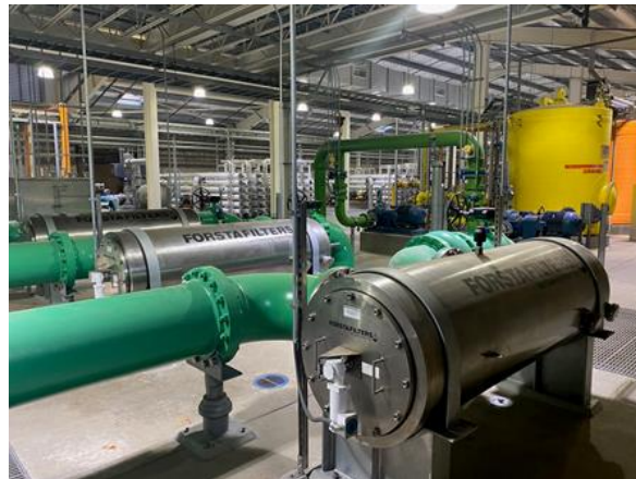
Figure 4 Forsta H18-LP180 Filters at Yucaipa Water Treatment Plant
