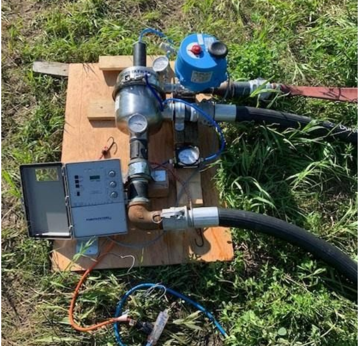
Forsta filter and backwash controller, the lower hose is the inlet, the middle one is the outlet and the differential pressure gauge is between them. The top (red) hose with the control valve goes to the backwash tub. The grey box is the automatic backwash controller.
