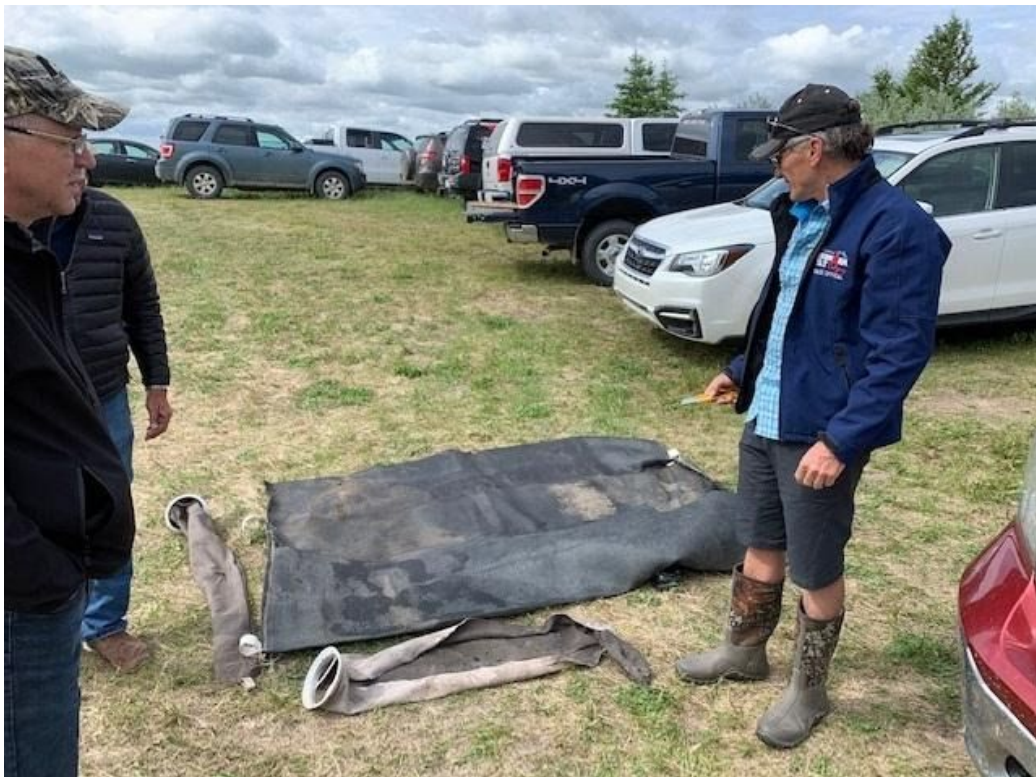
Inspection of the first Geotube and the downstream SOC filter after test run
