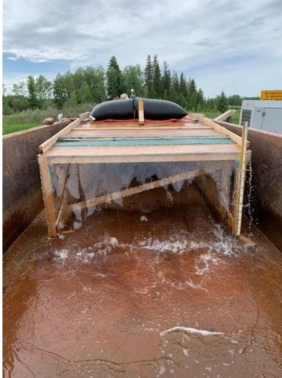
The inflated geotube being run at full flow rate of about 80 usgpm early in the test
