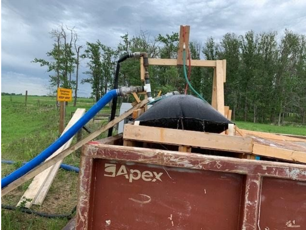
Final test configuration with a fully inflated geotube showing signs of pressure stress
