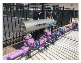
The filter was installed by a local contractor in the Spring of 2018. The filter has been operational and trouble-free for over a year and has required no maintenance since the initial installation. Operators have programmed the system to irrigate all of the campus landscape irrigation zones at one time. The landscape itself is evidence of the success of the system, and a glowing example of how reclaimed water can be used to make beautiful green spaces more sustainable.
