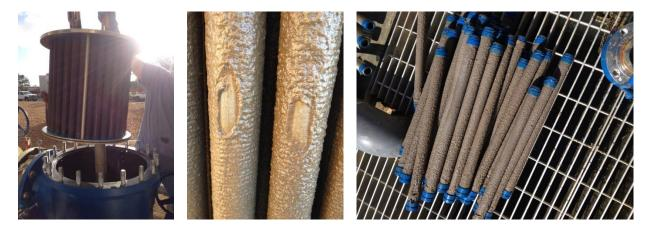
Once disassembled, the strainer candles had to be individually power-washed in order to resume system operation.
