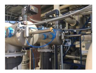
After the final material adjustments were made to the full-scale installation, equipment was monitored for a 30-day trial period starting 10/2/17. During the trial period, the bar for performance criteria was set at a 98% minimum recovery rate. The Forsta equipment exceeded the already stringent expectation by demonstrating a 99.9% recovery rate, and a consistent backwash interval of approximately 1x every 45 mins. The cleaning mechanism reliably relieved the differential pressure.
