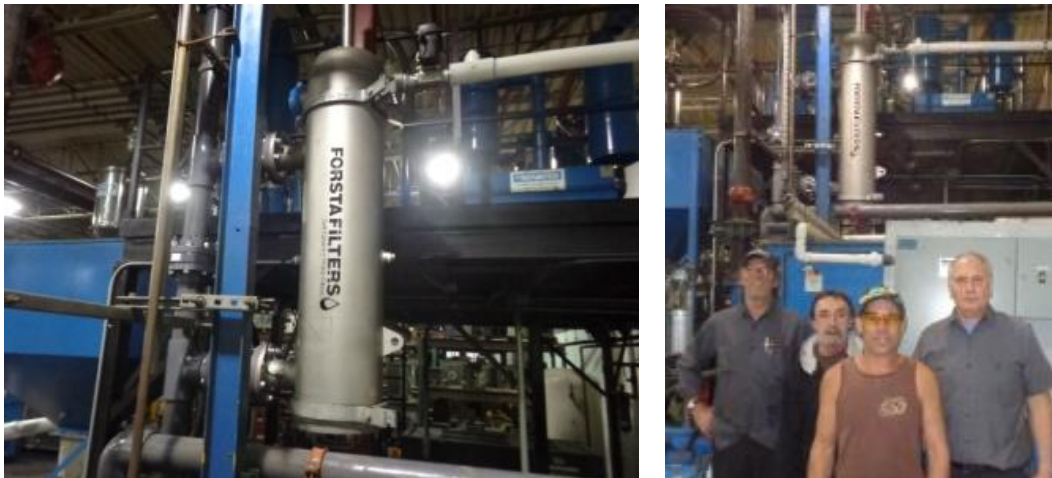
A team of 4 conducted the vertical installation at the Wolfeboro facility
