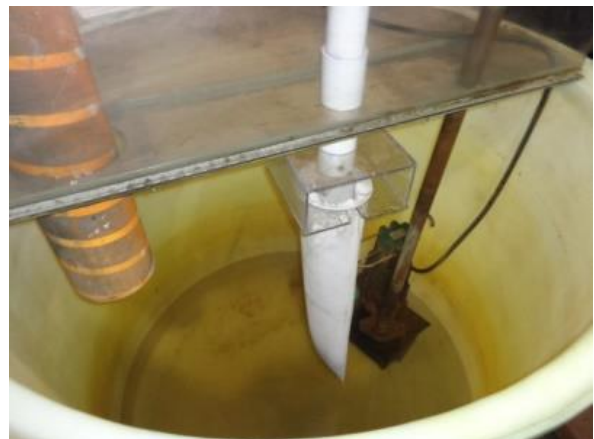
Backwash Water Recovery System
