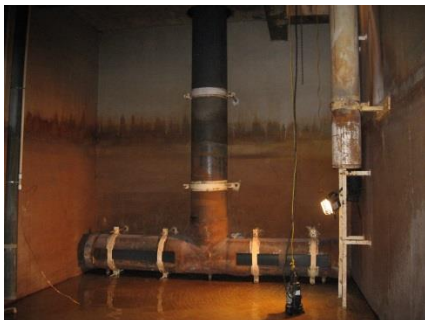
Inside view of the Coldwell
