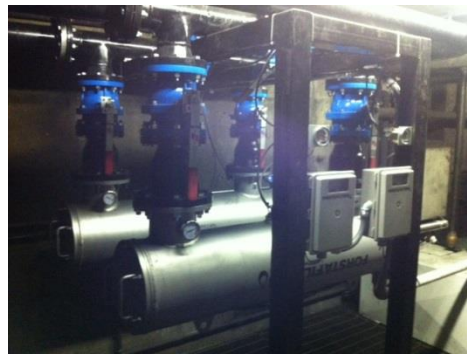
2x Forsta B6-180 model filters equipped with 316L high porosity 50 micron screens.
