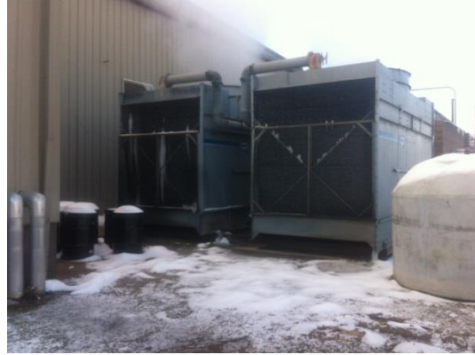
Superior's two cooling towers on the loop serviced by their Forsta self-cleaning filters.
