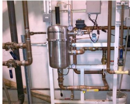
Forsta B2-90 model filter at the F.B.I. CJIS Division Facility. Filter is equipped with a 316L high porosity 100 micron screen.
