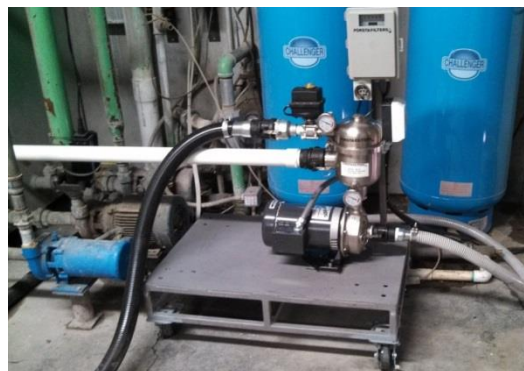
Forsta M2-90 skid mounted filter equipped with a 316L high porosity 50 micron screen, 50gpm pump, & 230/460 3 phase motor.
