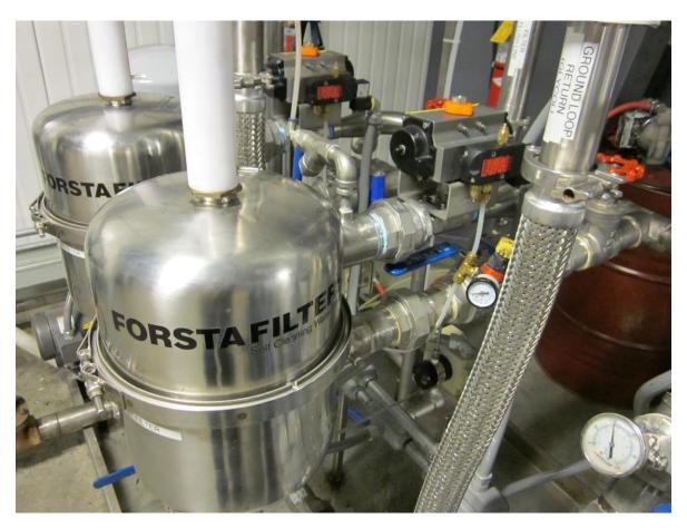
After contacting a number of different manufacturers, Michelsen chose Forsta because the company provided, "High quality units at a lower cost than the other manufactures." Bruskland said, "We also really liked the fact that the filter operates on inlet water pressure alone and does not require an external source of water for the very short backwash."
