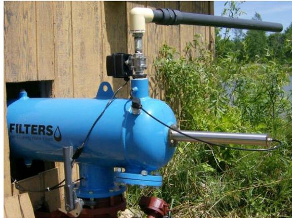
This is precisely what Marty Van Ells of Municipal Well and Pump was aiming to avoid by installing a filter in his irrigation project. Forsta self-cleaning irrigation filters provide insurance against costly landscape and turf damage, and prolong the life of sprinkler equipment. The automatic backwash cycle completely cleans the filter, eliminating the need for routine maintenance.
