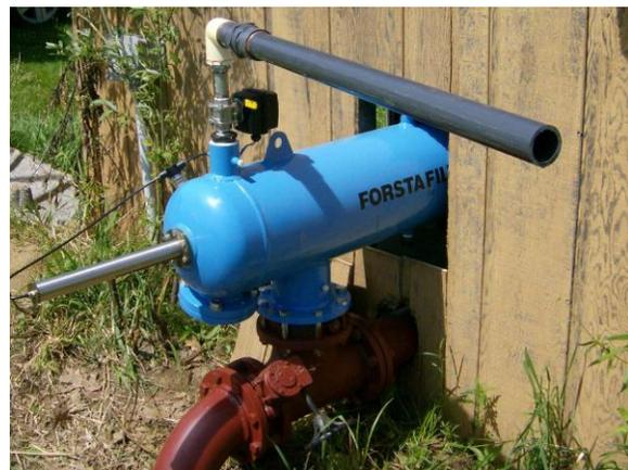
The filter, installed at the pump discharge, utilizes line pressure to complete its point-of-suction backwash cycle. This unique approach to backwashing ensures that even while cleaning itself, filtered water continues to flow. This also eliminates the need for standby filters and elaborate valve schematics, frequently needed with other types of filters.
